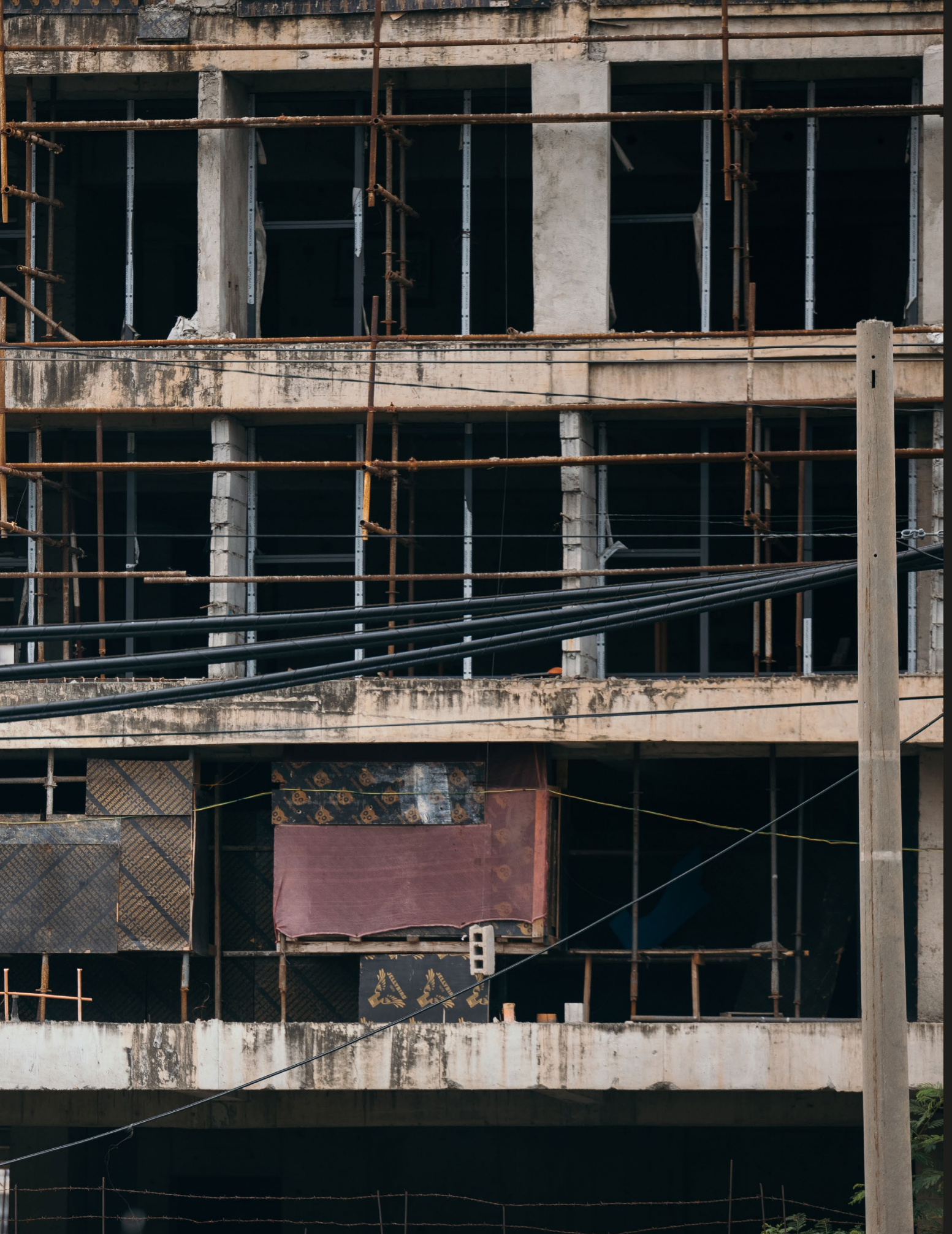
Workers taking a break at a construction site in Pasay, Metro Manila Philippines. The Philippines has seen a growth in property sales due to online gambling firms, aka POGOs (Philippine Offshore Gaming Operators). In recent times, President Bongbong Marcos banned all POGO companies due to the illegal activities including prostitution, money laundering, and abuse conducted inside the buildings.
