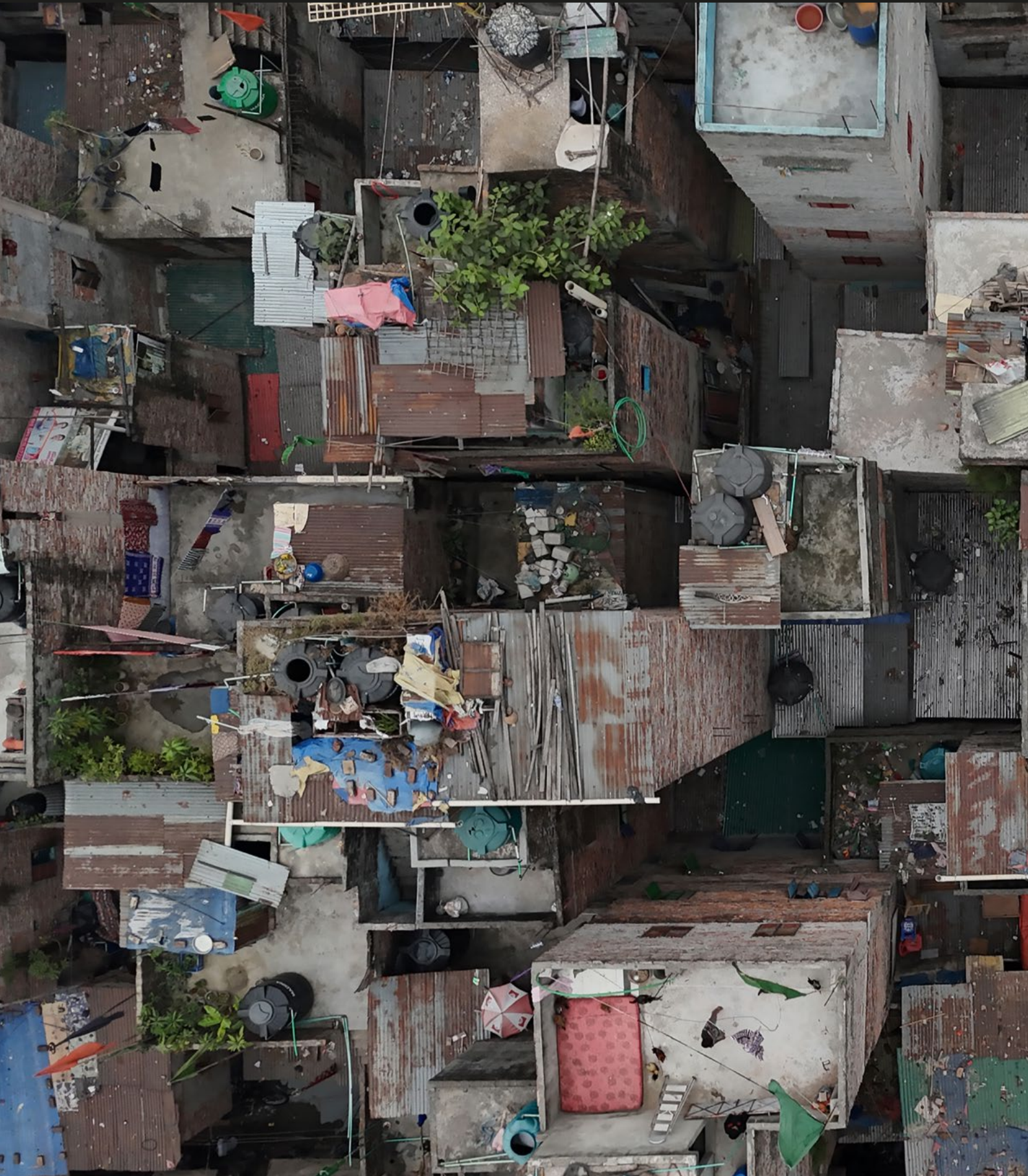
An aerial view of the homes inside Geneva Camp. Most buildings are made up of only two or three small rooms. All the buildings are less than 28 m 2 , a very limited living space for the families in the camp. Photograph by Naimur Rahman, 2025.
