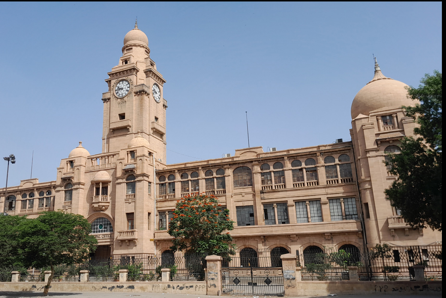
The Karachi Metropolitan Corporation (KMC) building. Photography by Wara Irfan
