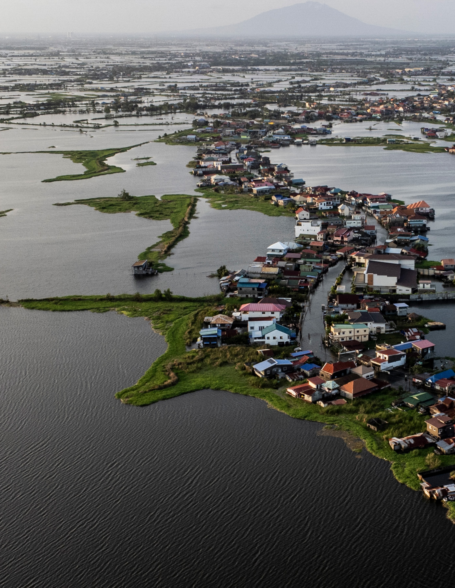
General view of the flooded houses following the typhoon Doksuri (local name: Super Typhoon Egay) and monsoon rains in Macabebe, Philippines, on August 5, 2023.
